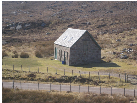
24 NG 84499 54414 23m ruined house/barn
